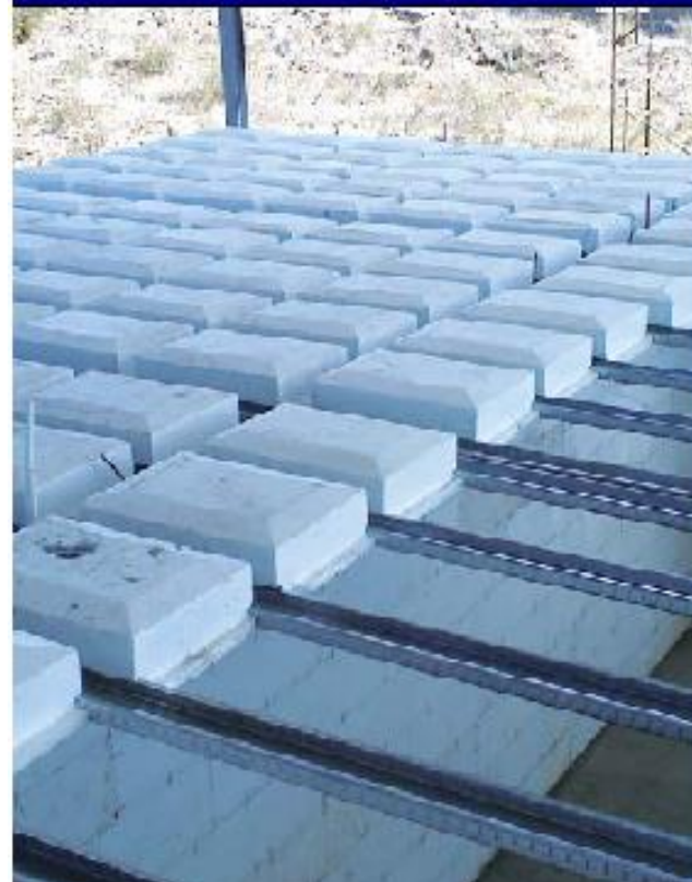
TASS slab in progress
