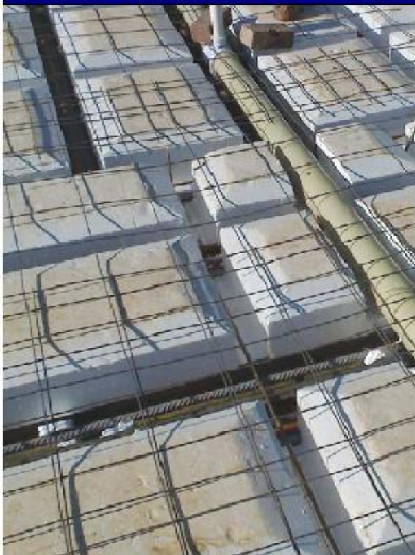
Easy installation of services into a TASS slab
